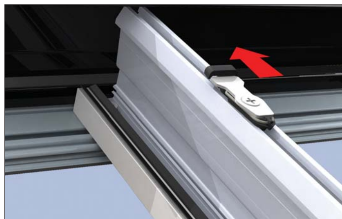
Ensure the clip is orientated as shown, with 'trigger' towards the ridge.
