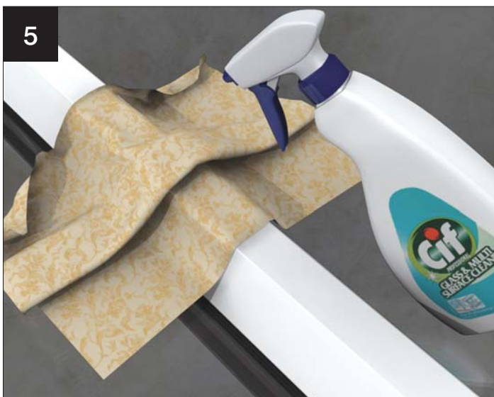
5 Stubborn marks can be removed using a renovating cream like CIF or perhaps T-cut. Once dry, buffing can take place.
